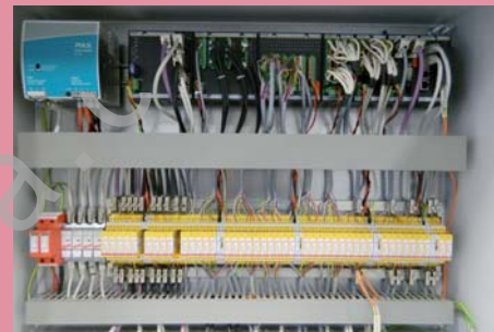
▲ A match for all weather: The Bachmann M1 controller in the lightning protection laboratory
